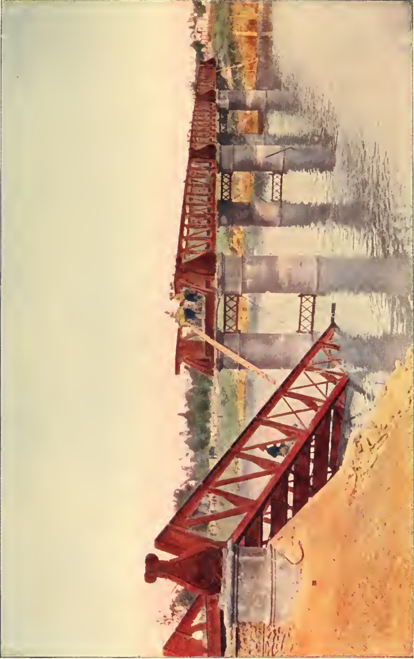
Railroad bridge over the Bagbag river partly destroyed by insurgents to prevent the Americans from crossing. Insurgents guarding the bridge were forced to retire and the engineers' corps built steps for the troops to cross and assault the enemy beyond.
